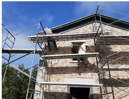
Scraping Cornice Trim before Repainting
