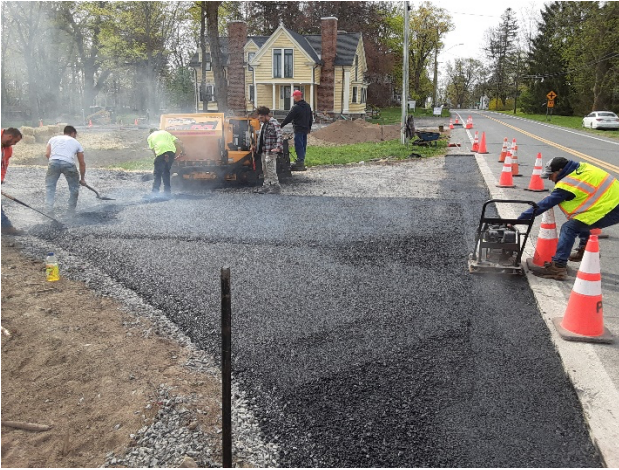
Asphalt Highway Approach being placed
