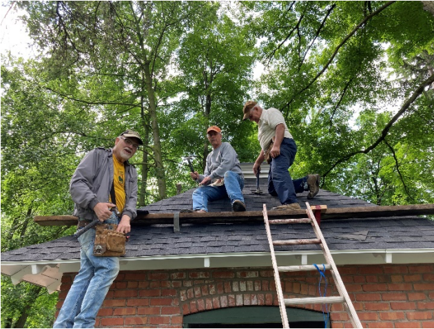
Larry Bell, Guy Garnsey and Gus Littlejohn Installing shingles
