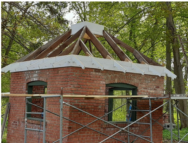
Roof Framing with Scrolled Outlooks on Rafters
