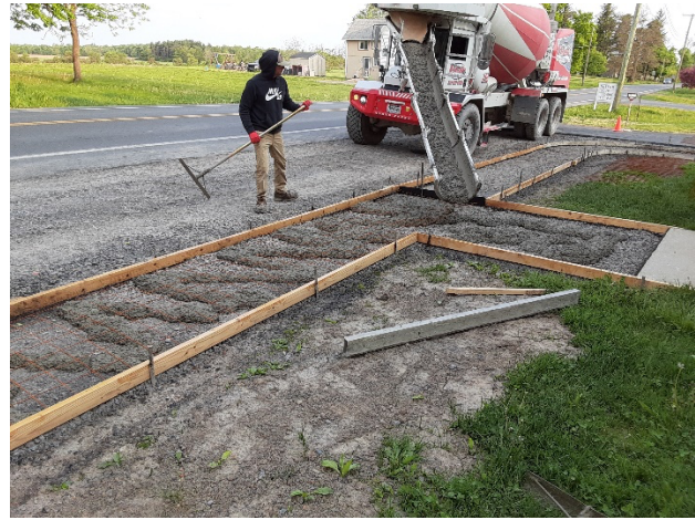
Sidewalk Concrete being poured
