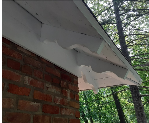
Refabricated Historical Rafter Outlookers
