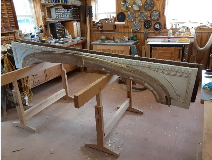
Hallway Arch being restored
