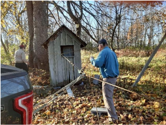
Historic circa 1830 Outhouse being lifted up on temporary foundation
