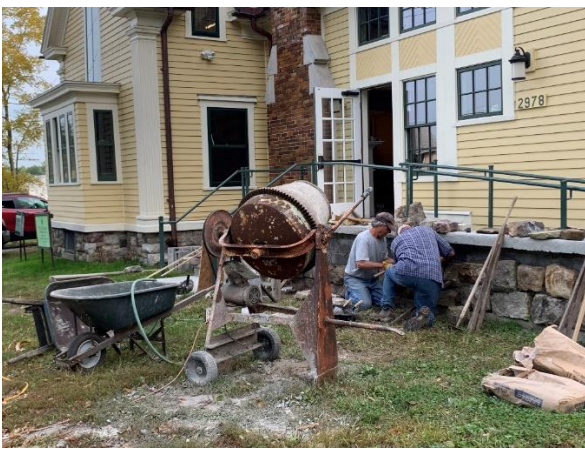
Stone Veneer installation on Handicapped Ramp
