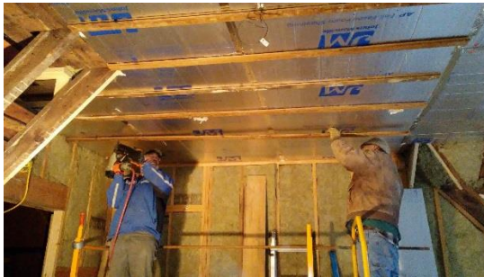
Archive Room Insulation
