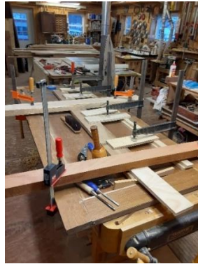
Historic wood veneer doors from North Wing which were badly damaged by moisture being refurbished.
