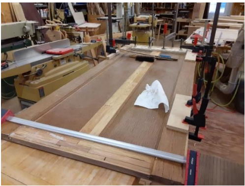
Historic wood veneer doors from North Wing which were badly damaged by moisture being refurbished.
