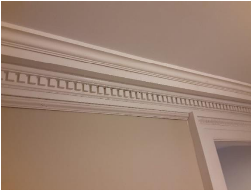
Refurbished historic crown molding in entry Hall.
