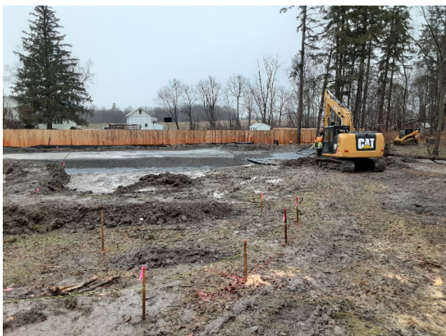
Grading and Stone Fill
