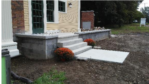
Front Stairs and Accessible Ramp
