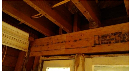
Replaced French Door Header
