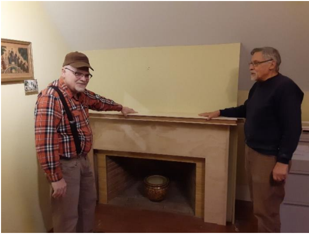
Gutchess Mantel carcass in position
