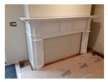
The salvaged mantel from the demolished south wing has been completely restored and relocated to the Entry Hall.
