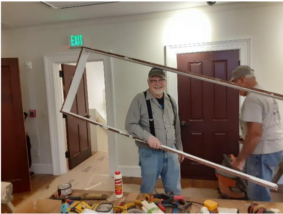
Larry Bell working on door frames
