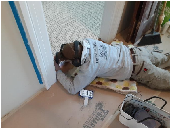
Andy Simkin installing floor tile
