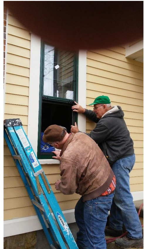
Storm Window Installation Larry Bell and Gus Littlejohn
