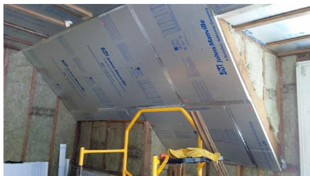
Polyiso Boards Installation
