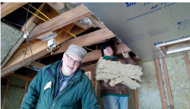
Rockwool Installation
