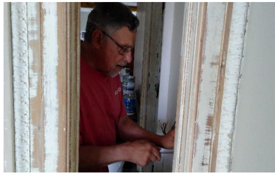
Volunteer Tryg Ager installing electrical light switches
