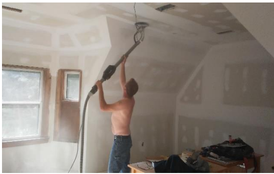
Drywall finish sanding
